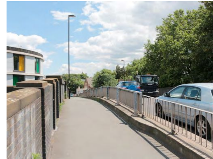
Railway and Ravensbourne River create east-west severance, navigated by the tall highway bridge. Potential to improve crossing access and cyclability.
