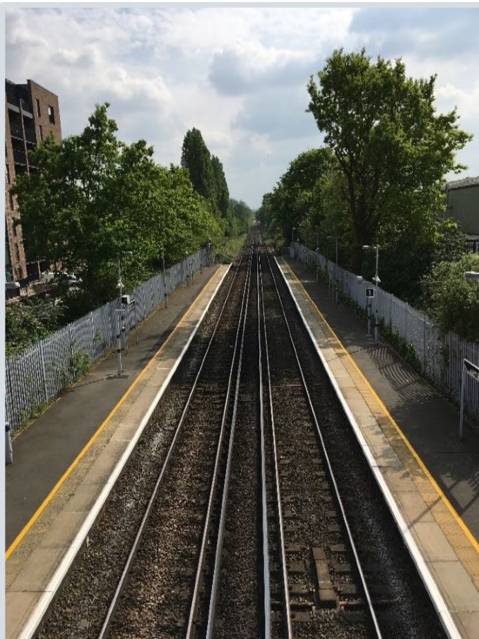
Lower Sydenham station
