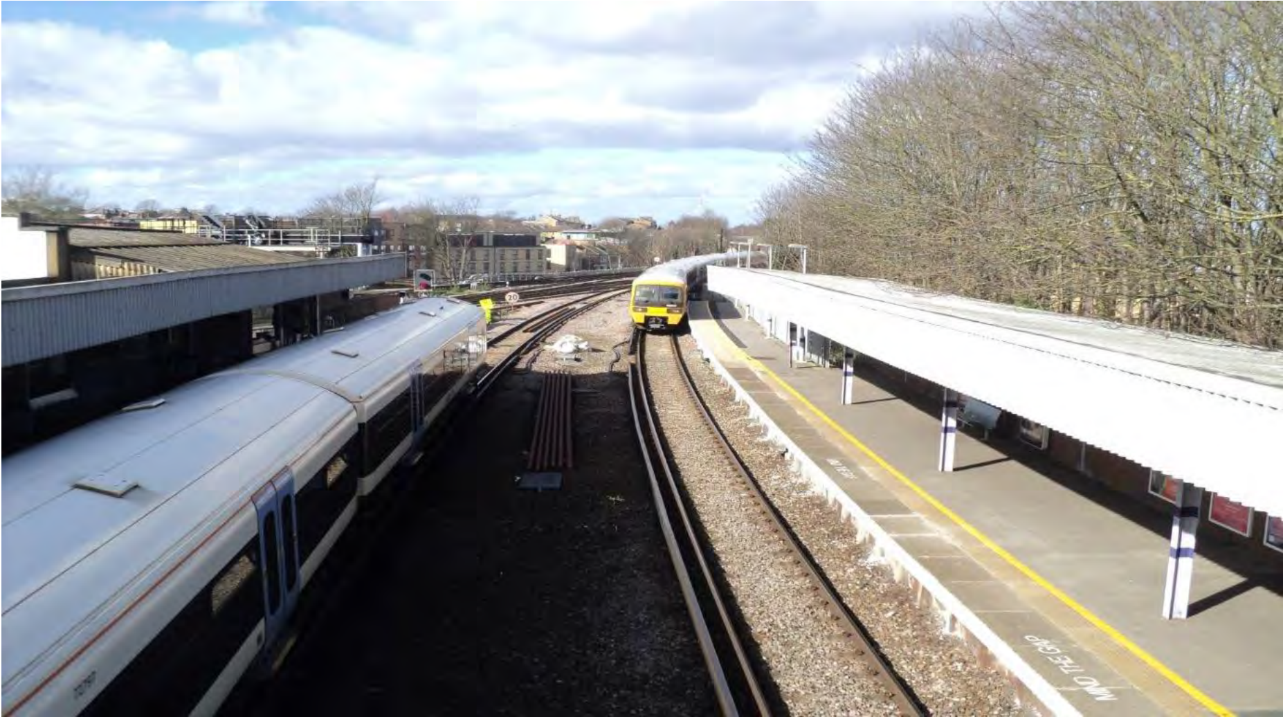
Trains crossing at Hither Green Railway Station, on the London Charing Cross/Cannon Street to Sidcup and Orpington Lines
