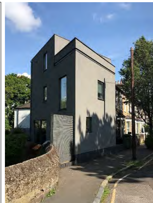
Right. Weardale Road, Lee Forum area. New build house's sharp geometry, accentuated by contrasting render to the adjacent Victorian terrace, is defined by challenging constraints of the infill site, with its riverside location. Fenestration is limited and playful. Setting point lines with frontage of adjacent terrace, and a relief line in the render with adjacent eaves. Top floor is set back to reduce its impact on the street scene. 31/44 Architects
