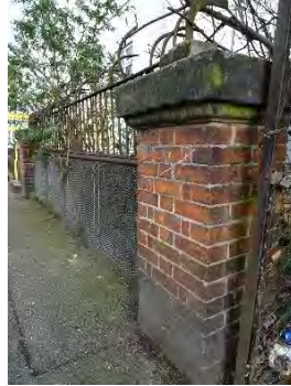
Bridge, Eastdown Park
