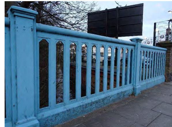
Bridge over River Quaggy, Lee High Road
