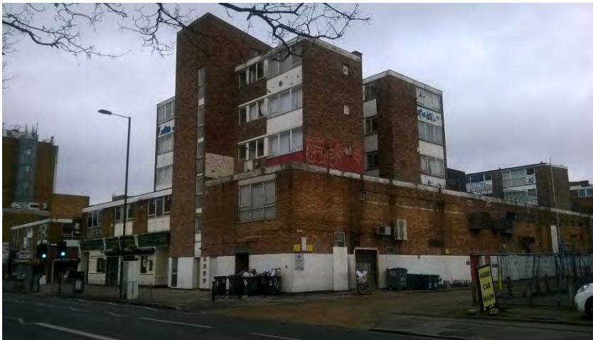
Leigate, Burnt Ash Road
