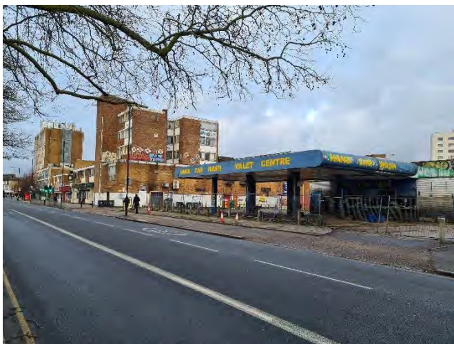
Leegate Shopping Centre, SA10
