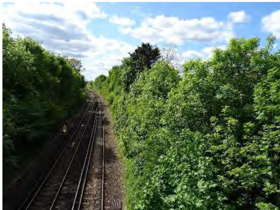
Railway tracks, from South Circular bridge
