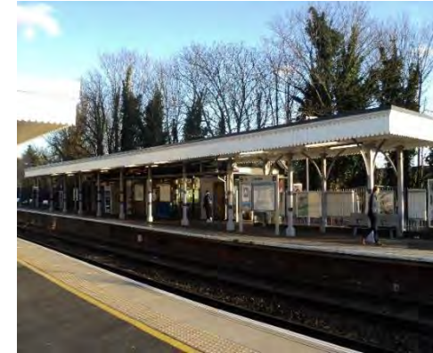
Platform 1, Lee Railway Station
