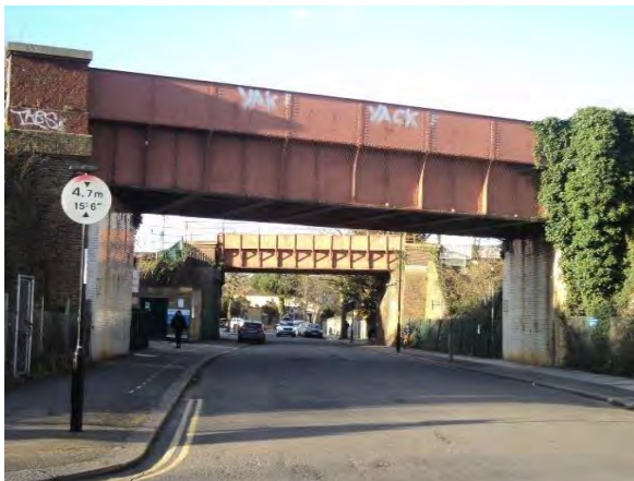
Two railway bridges at Manor Lane
